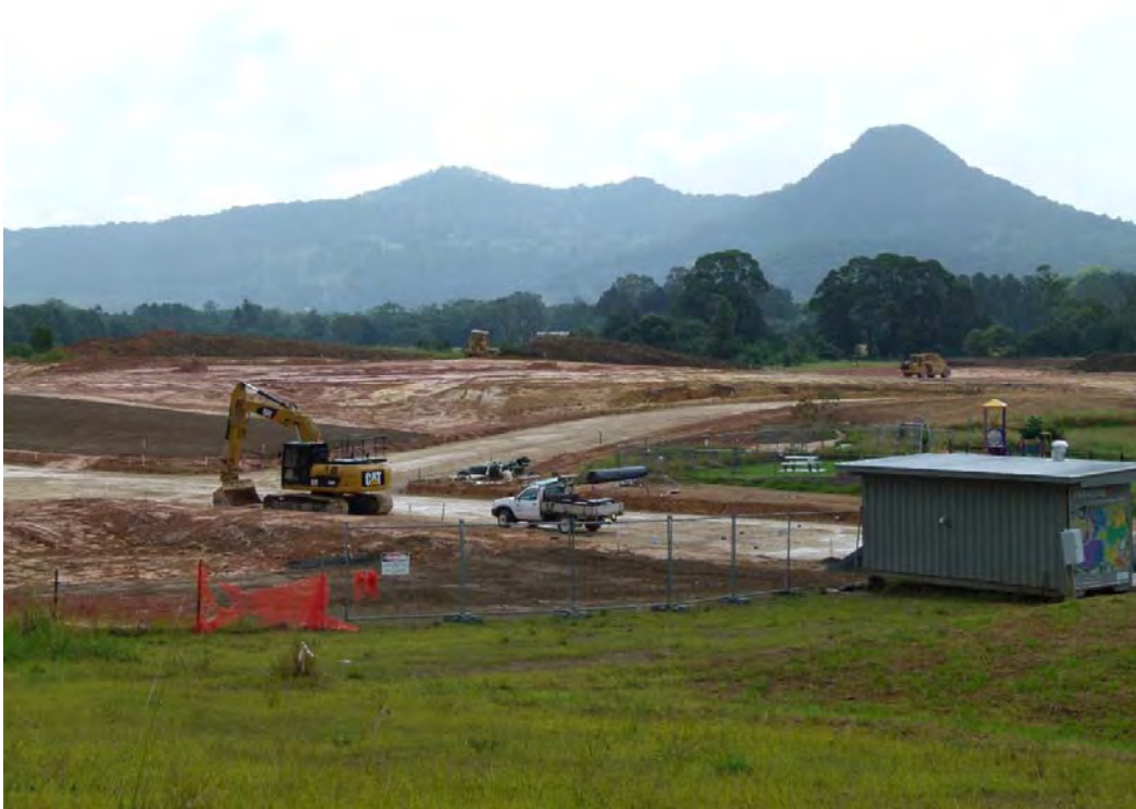
Plate 4: Development of Stage 2 at the Tallowood Ridge estate
